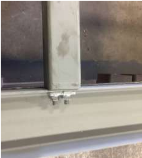
Figure HP-1 Half Post Connection to Channel
